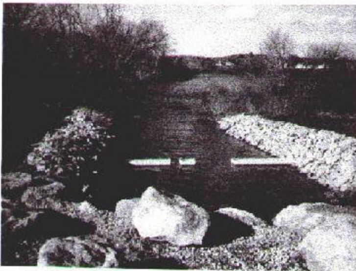
The finished weir and newly stone-fortified banks
