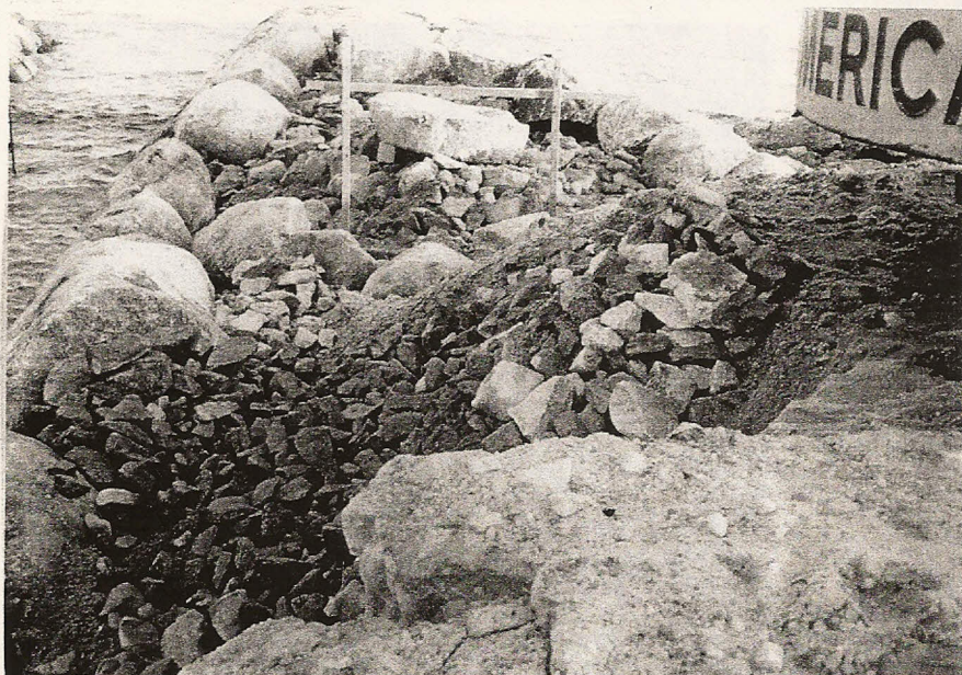
Anatomy of a Jetty: Construction Work Winter 2001
