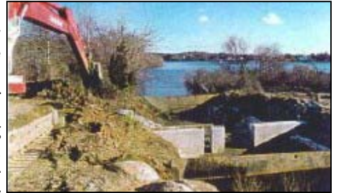
Construction of the weir in 1998. Photo R. Livingstone to everyone.
