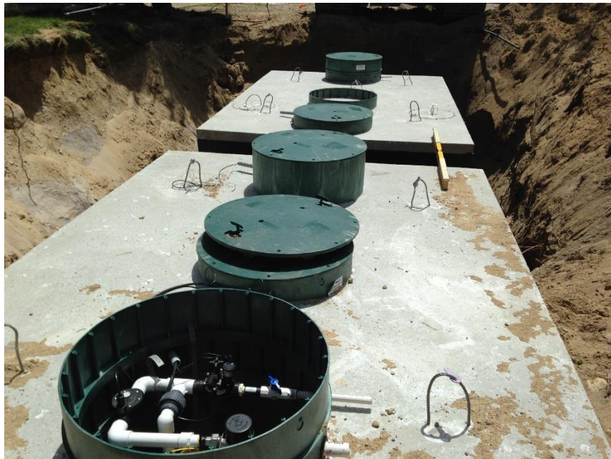
Hoot system installed as part of a full upgrade from cesspools at the location of Case Study HO2.
