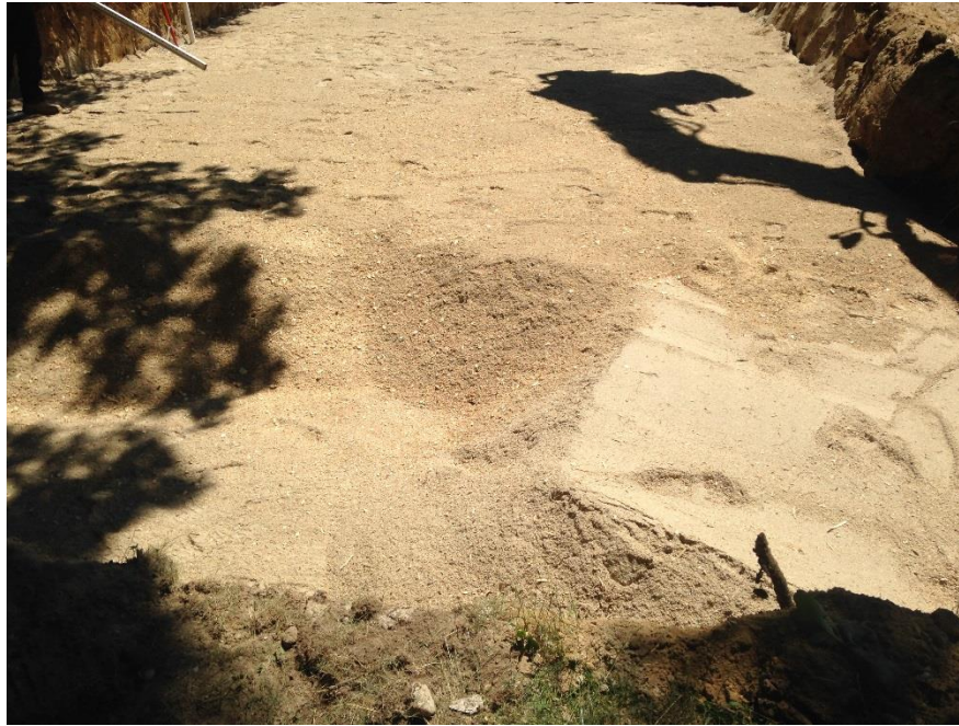
Layered STA installed as part of a full upgrade from cesspools at the location of Case Study #6.
