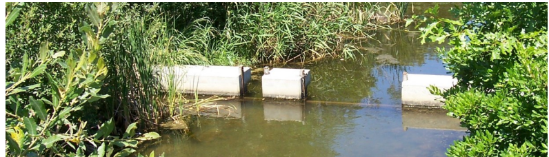
The adjustable weir in Trunk River can be used to control water flow out of Oyster Pond.
