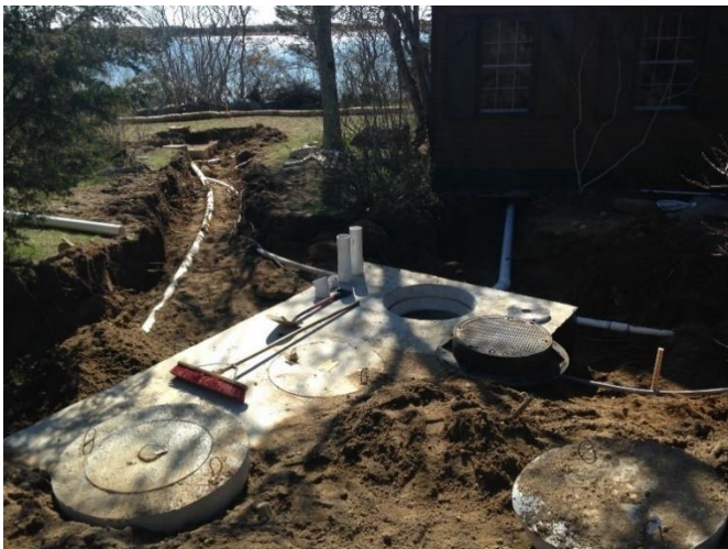
2,000 Gallon Blackwater Tank installed in parallel with an existing Title V systems at the location of Case Study BW9.
